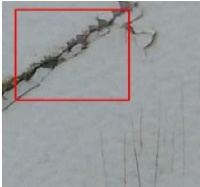
**Figure 6: Crack detection result shown with bounding boxes [57]**
