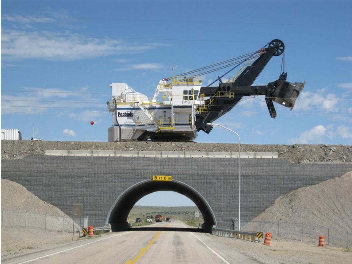
**Fig. 2-1: Large-span soil-steel structure in Grants, New Mexico (after Hahm, 2021)**
