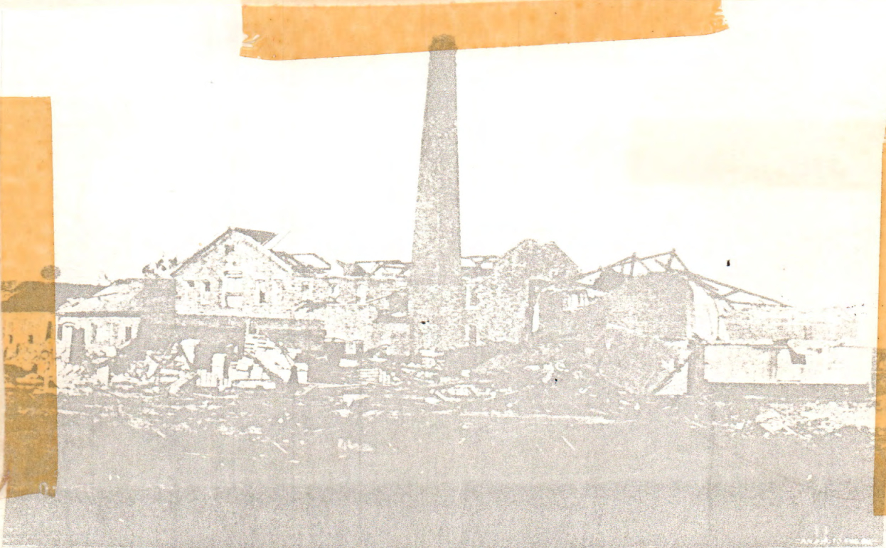
MERRITTON TORNADO.—THE LINCOLN PAPER MILLS, SHOWING THE WRECK OF THE ROOFS OF THE VARIOUS BUILDINGS AND THE WALLS OF THE STOREHOUSE. IT WAS HERE THAT MISS CLARA O NEAL WAS KILLED AND MANY OTHERS INJURED.
