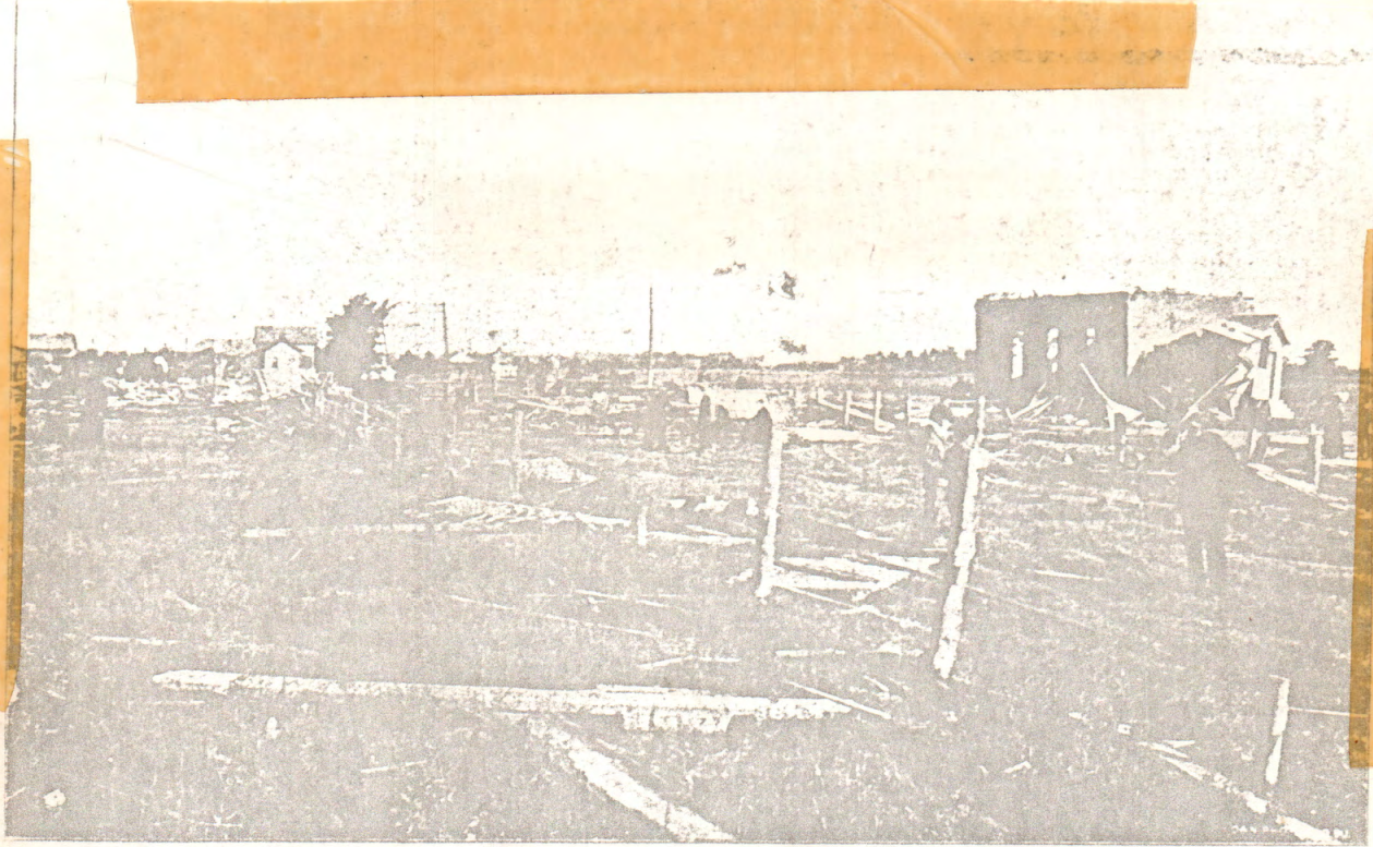
THE MERRITTON TORNADO. SCENE AT THE LOWER PUBLIC SCHOOL, WHERE LITTLE FRANCIS MOFFATT WAS KILLED. THE WALLS OF THE SCHOOL ARE STANDING. THE DEBRIS IS ALSO SHOWN OF THE ORANGE HALL, AND OF J. E. BRADLEY'S HOUSE, IN WHICH MRS. BICKLEY WAS KILLED. BOTH THESE BUILDINGS ARE COMPLETELY LEVELLED.
