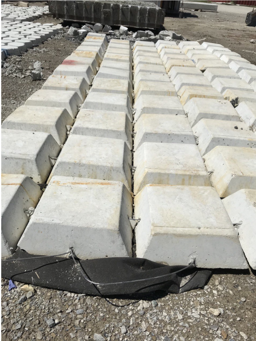
Figure 3.8: Blocks with geotextile attached (Credit: IECS Inc)
