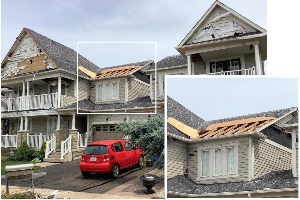
**Figure 10: Roof sheathing failure on gable roof from Barrie tornado on July 15th, 2021, photo courtesy of Northern Tornadoes Project**
