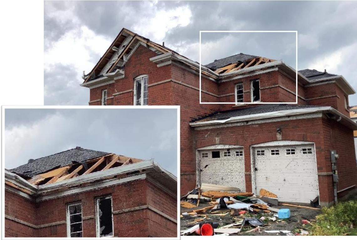
**Figure 9: Roof sheathing failure on hip roof from Barrie tornado on July 15th, 2021, photo courtesy of Northern Tornadoes Project**
