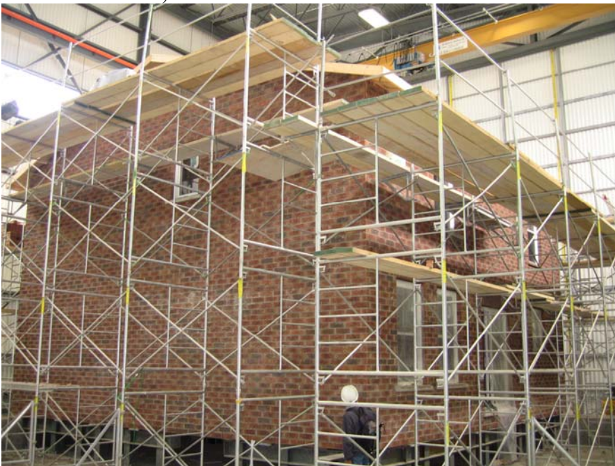
a) Full scale test house during construction (Modification has been made to avoid commercial issue.).
