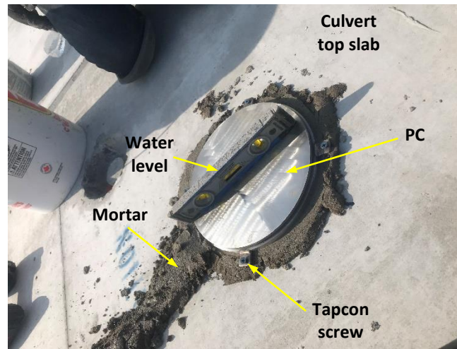
Figure 3-8. Pressure cells installation on the top slab of the Remembrance culvert.
