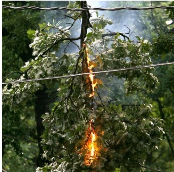
Figure 1.1: Arcing ignition caused by power lines touching tree branch.
