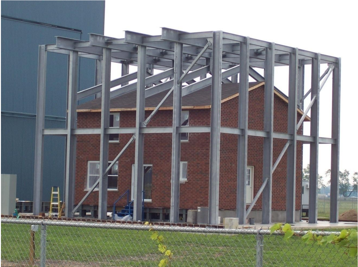
Figure 2.1 Photograph of the test house surrounded by the steel reaction frame used to mount the air bags and PLAs.
