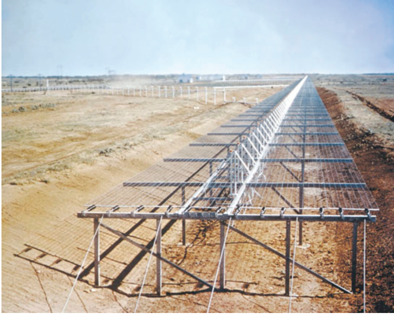
Fig. 4. Air force space surveillance system, part of the master transmitter antenna at Lake Kickapoo, Texas, c.2001. Photograph by an employee of the United States government. Creative commons public domain image.
