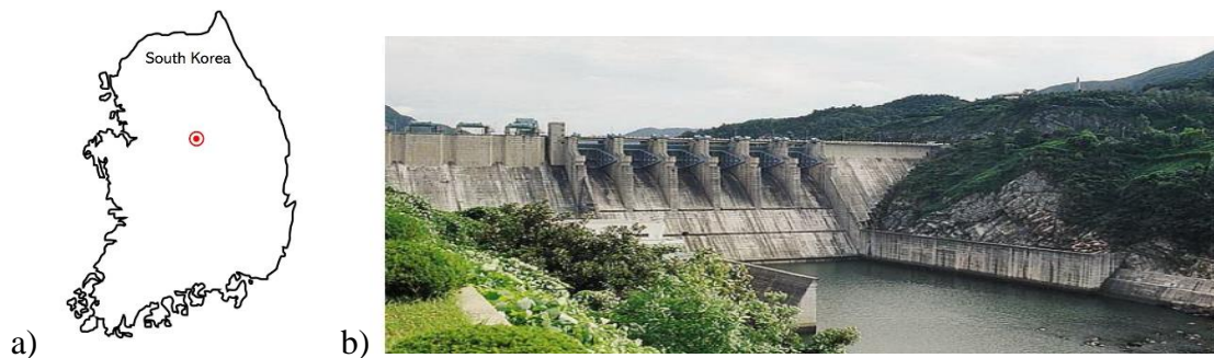
Figure 4.1: Location of Chungju Dam and a photo of the dam: (a) Location of Chungju dam, (b) photo of the dam.
