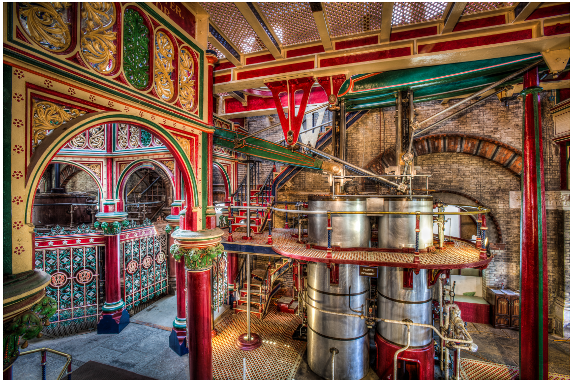
Figure 1: Photograph © Peter Scrimshaw 2012, taken of the Crossness Pumping Station, which was restored in 1987 and has since been maintained as a museum by the Crossness Engines Trust. Reproduced with the permission of the artist.
