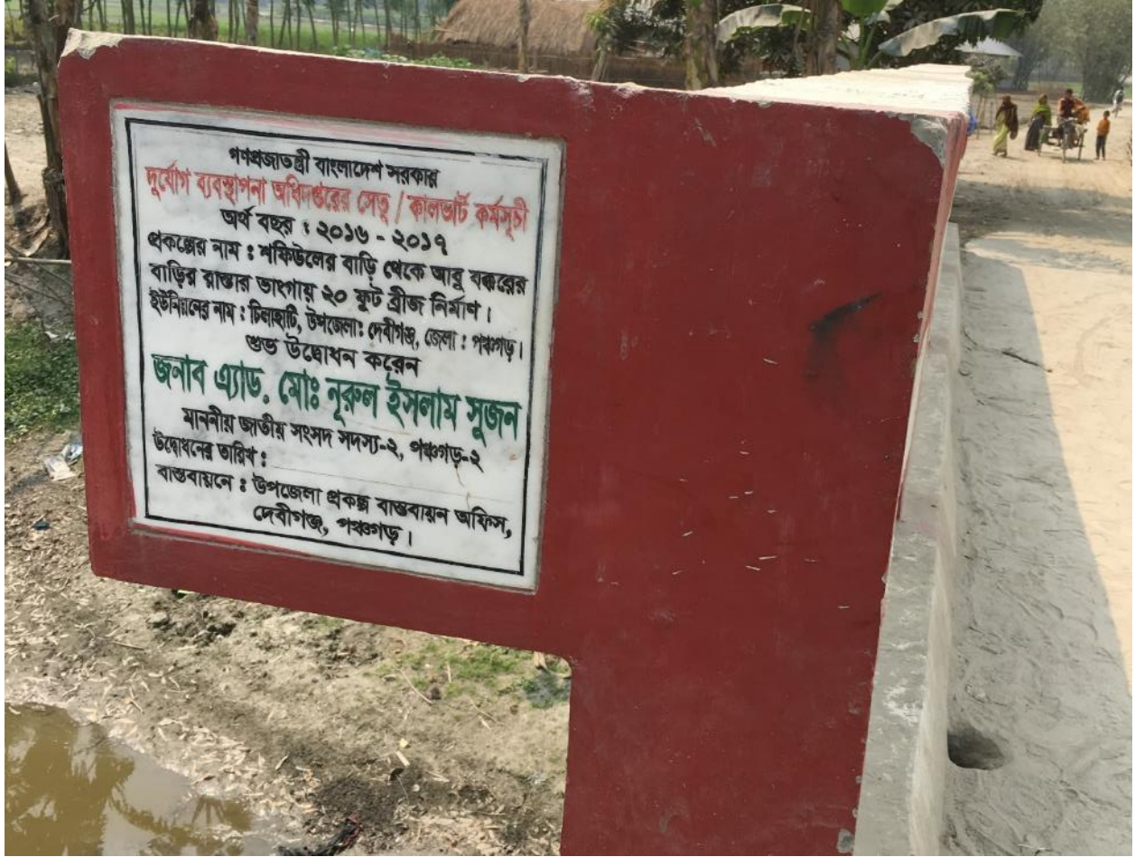
Figure 20: MP's name engraved in the newly built culvert in Balapara Khagrabari
