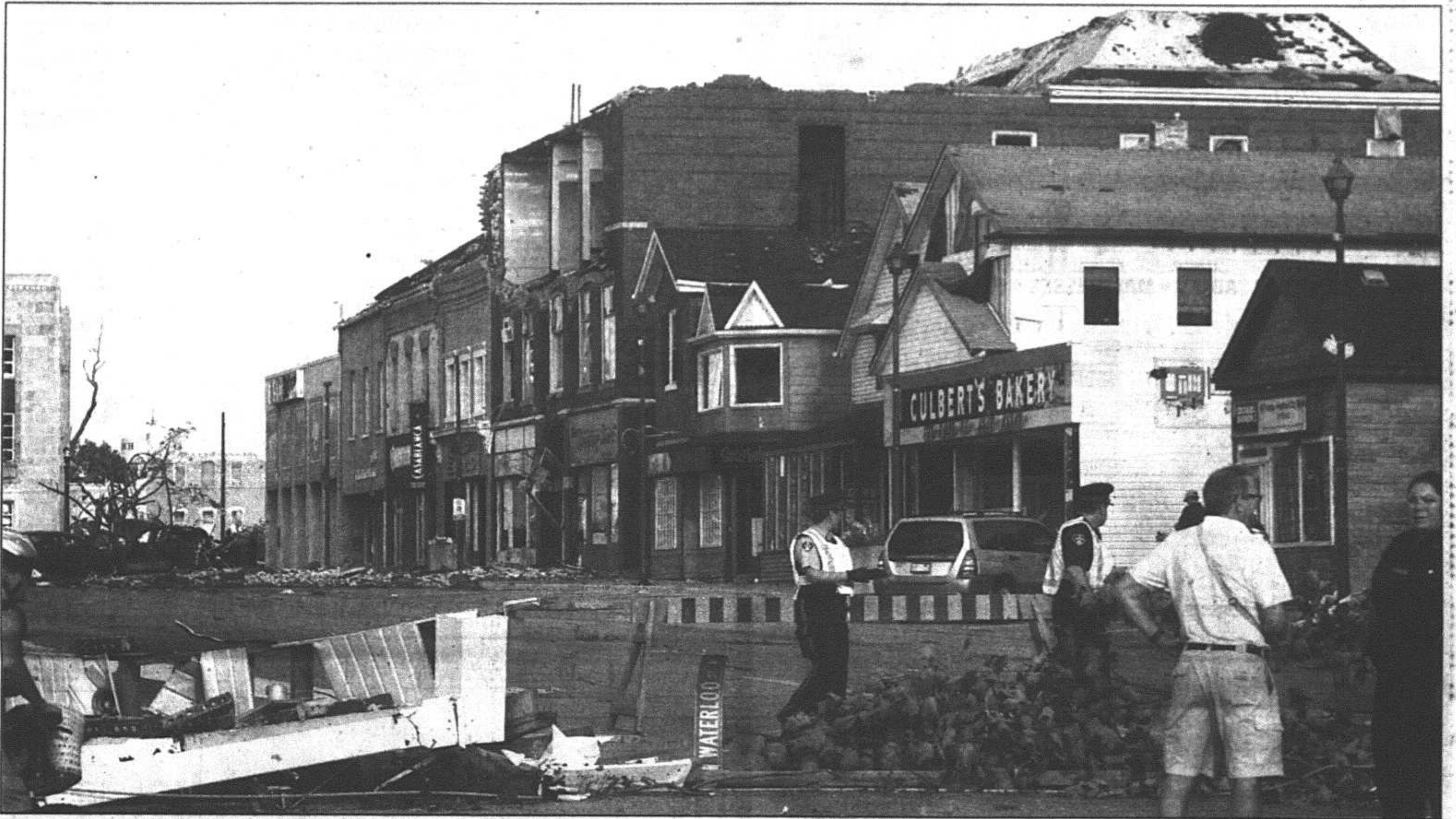
Buildings around Goderich's historic Square were heavily damaged when a suspected tornado touched down about 4 p.m. Sunday.
