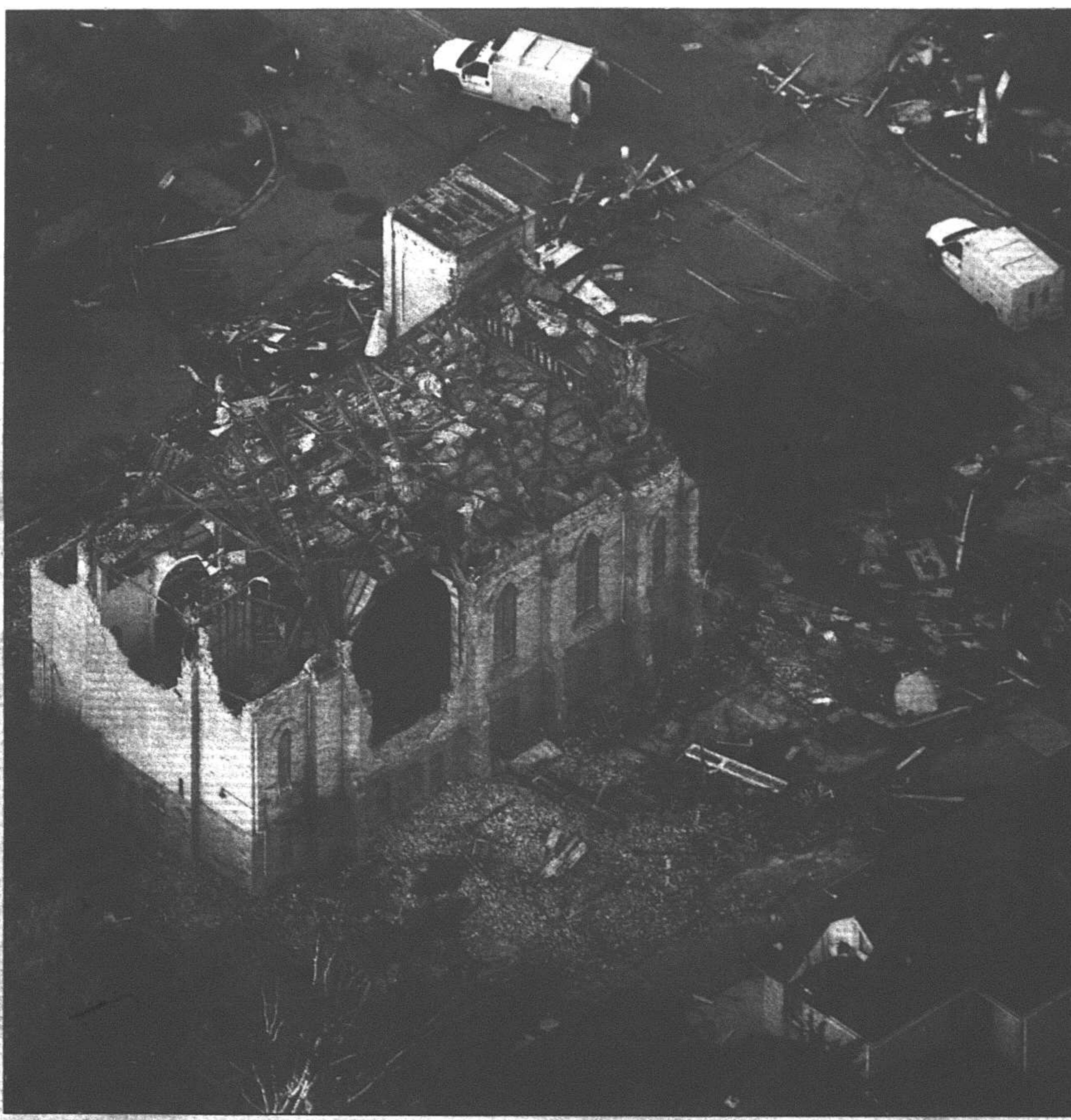
Victoria Street United Church stands in ruins after a severe storm ripped through the heart of Goderich Sunday afternoon, overturning vehicles, ripping off roofs and sending the picturesque lakeside community into a state of emergency. Early reports indicated injuries, but no fatalities, among area residents.
