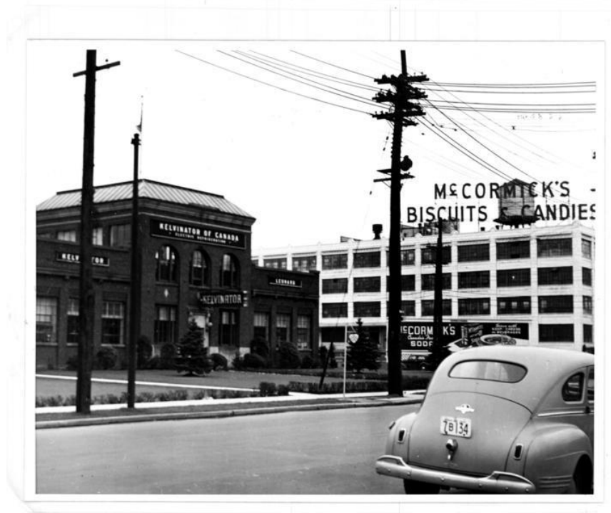
Figure 2.6 The McCormick's Factory in London, ON was purchased by the city and proposed out to private developers in the hope for its successful reuse (Ivey Family London Room, Central Library, London Public).
