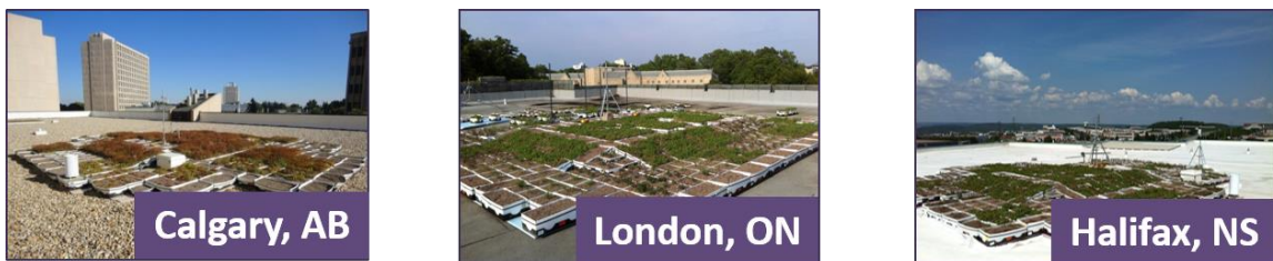
Figure 1: Site layout of the experimental modular extensive green roof at the three study sites.
