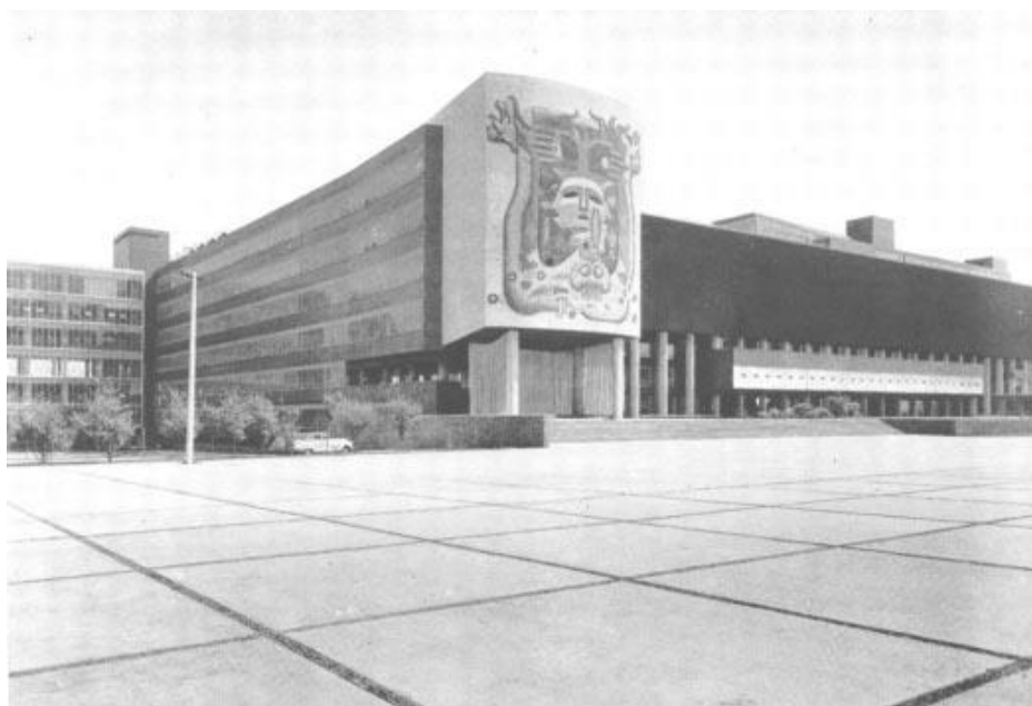
Figure 12 - One of the University of Mexico buildings where contestants in the Pan-American Games were housed and fed. 44
