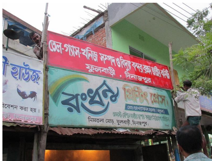
Figure 12: Installing signboard for new office space
