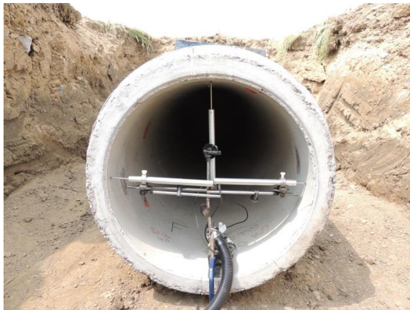
Figure 5-1 Pipe segment instrumented with LVDTs.
