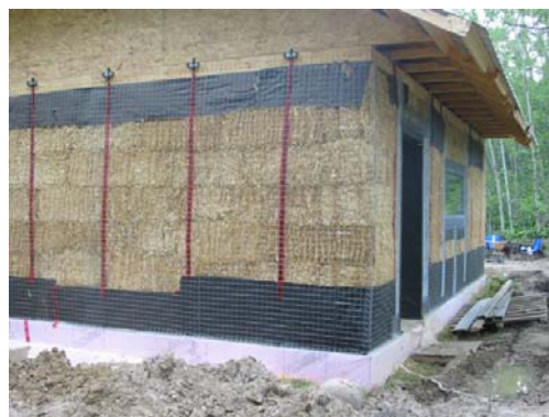
Figure 5-1: Straw Bale House in Construction
