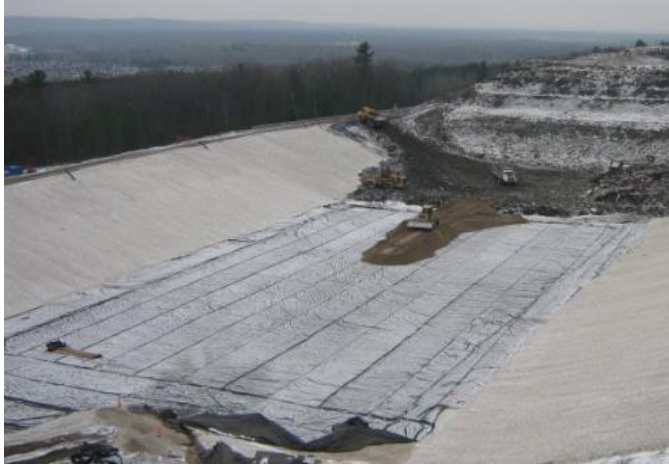
Figure 4: Construction of lined waste cell
