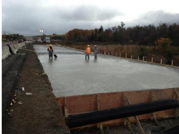
Figure 4: Geogrid Installation
