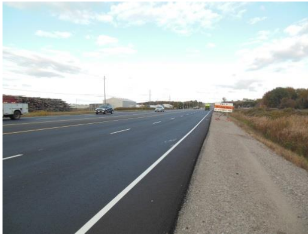
Figure 6: Completed pavement incorporating LFCF
