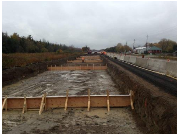
Figure 2: Excavation and Base Preparation
