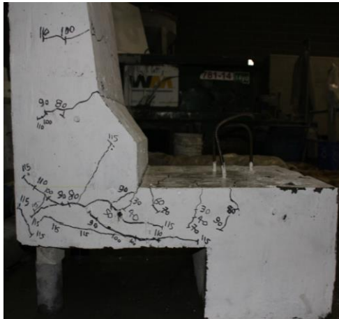
a) Crack pattern at the left side of the specimen
